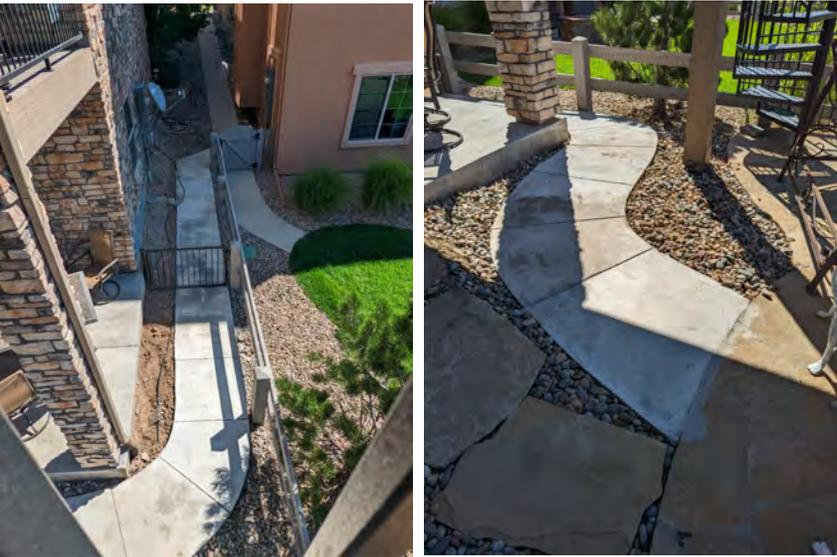
Pictures #5, 6 & 7 – These pictures show a more close up look of the grading on both properties and how they still slope towards the center after the sidewalk was completed. In the center photo, you can see how the neighbor's "old" sidewalk is tilted towards Norvel's property so that water would run off towards the center.
